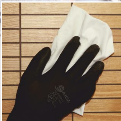
6. Once the grout has dried, clean the tiles with a damp cloth and polish them using "KERAKOLL FugaSoap@Eco".
