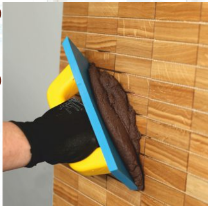
3. Apply the grout from bottom to top and across the seams.
