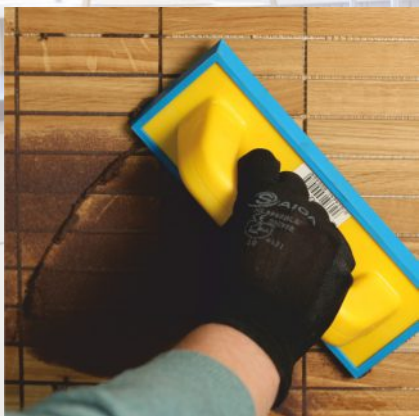
4. Spread the grout so that all the spaces get filled in evenly.
