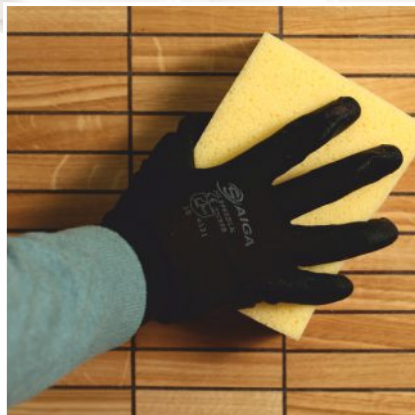
5. Clean the residue with a damp sponge. Use warm water to dampen the sponge.
